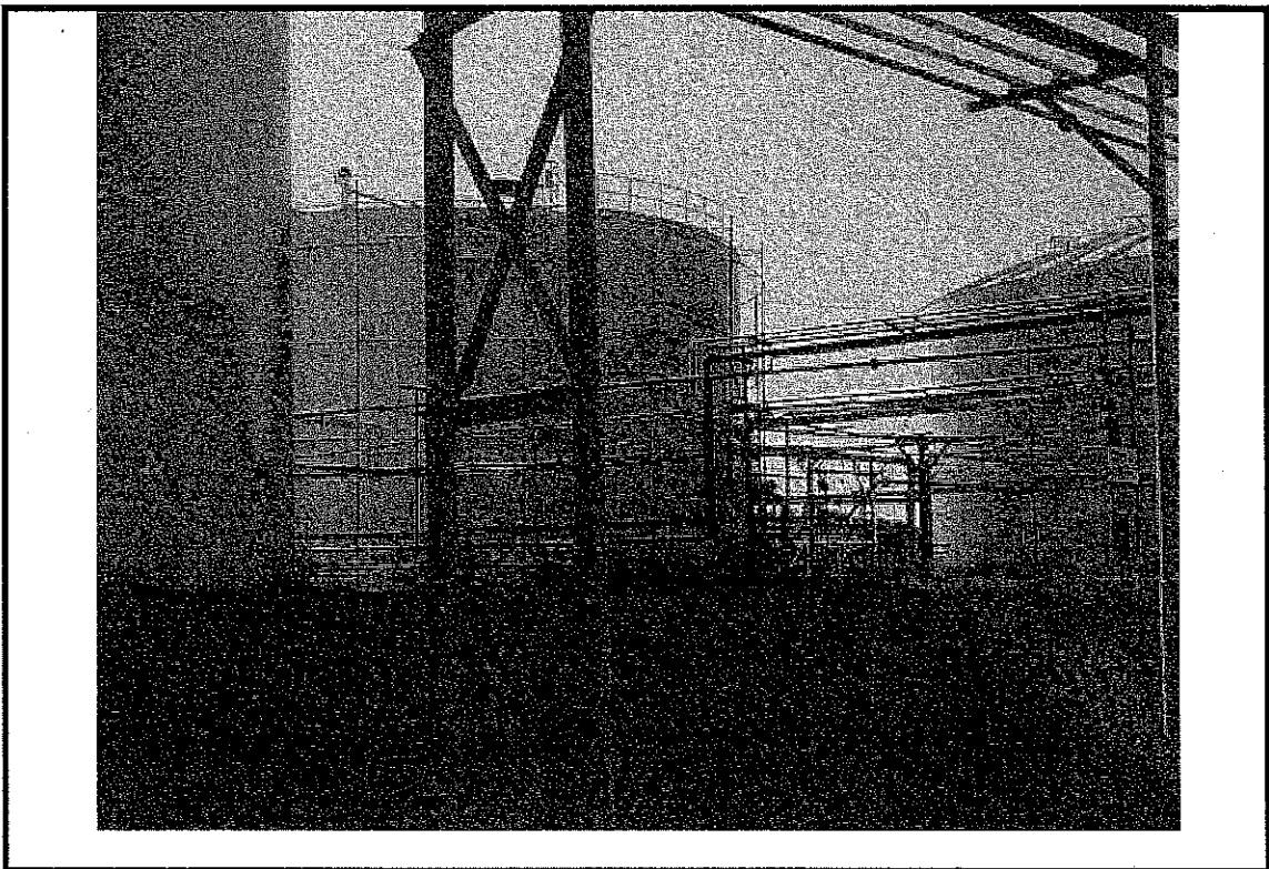
Photo 20: View of Styrene Tank Converted to Firewater Tank. View to Southwest.
