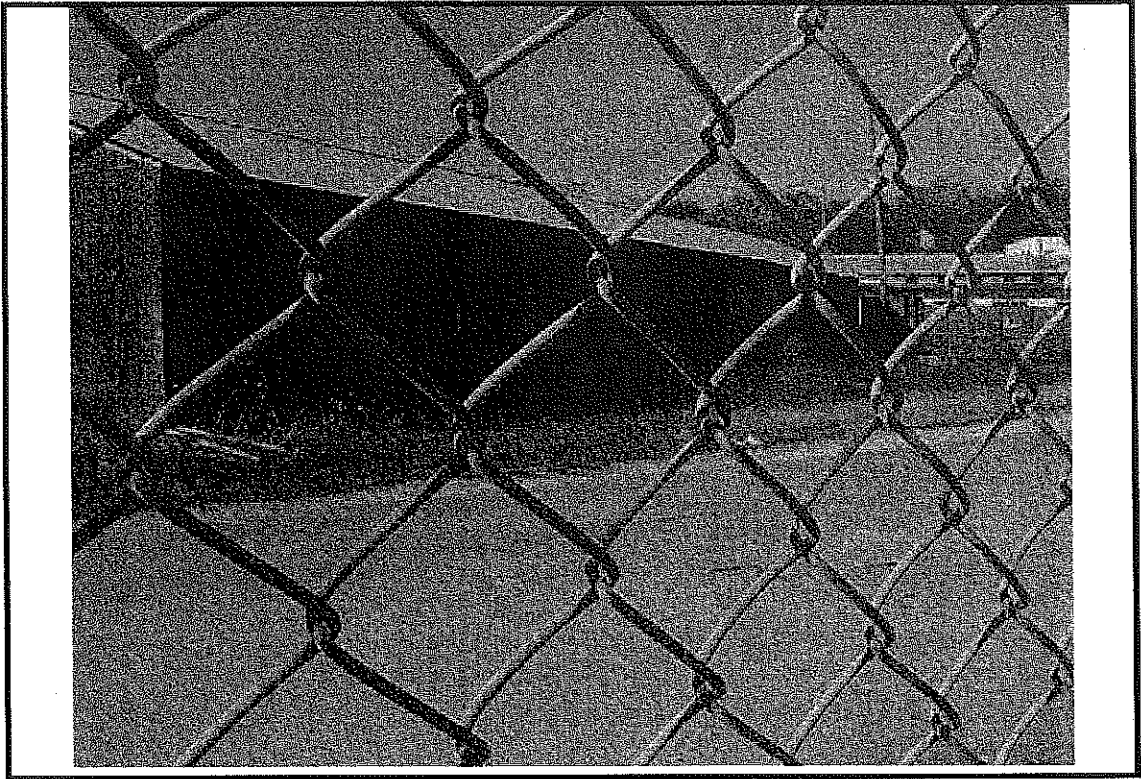
Photo 17: View of Godan Property Facing Northwest
